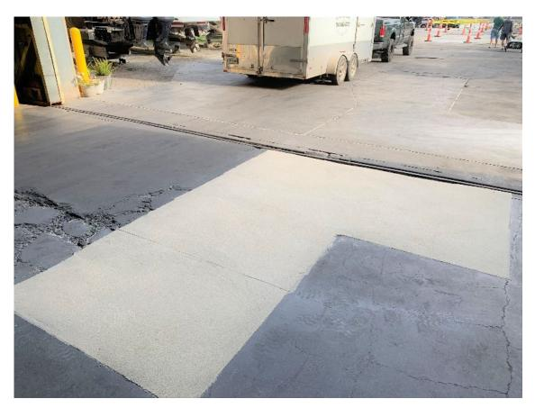
Mix 3 parts aggregate (sand, color quartz, aluminum oxide, etc.), with 1 part catalyzed FlexKrete,
